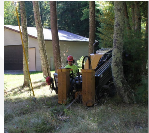
Directional Boring in a sensitive area
