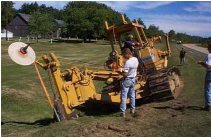
Plowing Method of Installation
