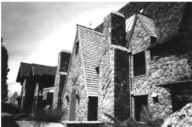
The cost of maintenance for the aging structure on the Thunderbird Lodge estate is conservatively estimated at $300,000 per year. OIG photo.
