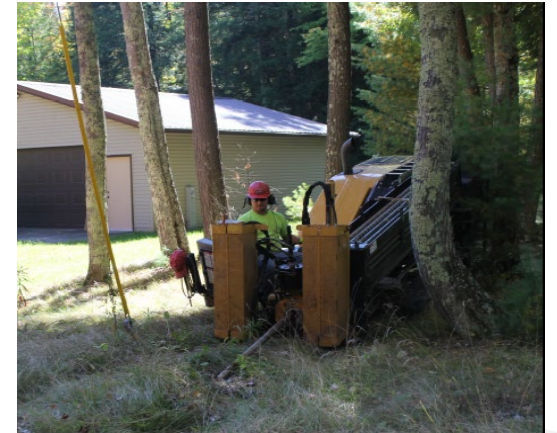
Directional Boring in a sensitive area avoids significant environmental effect
