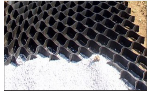
Cellular confinement panels being backfilled with gravel
