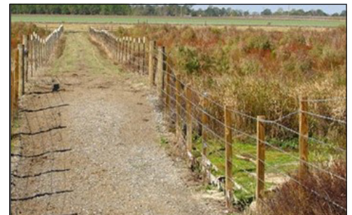
Fencing restricts livestock access to the crossing
