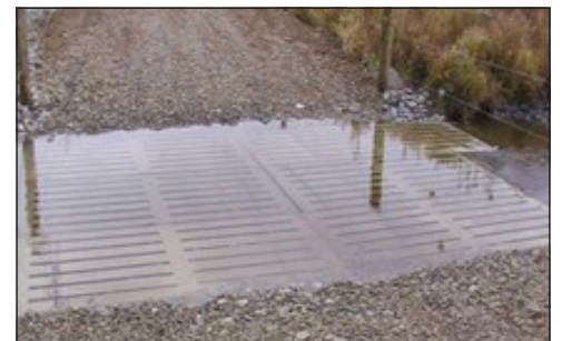
Hog panel stream crossing
