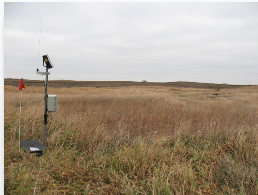
A view of an installed bioreactor, showing the upper control structure and warm season grasses that have re-established in soil covering the bed of wood chips in which water is treated.
