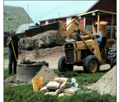
Well decommissioning requires professional help.
