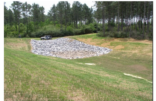
Rock Chute at end of waterway.
