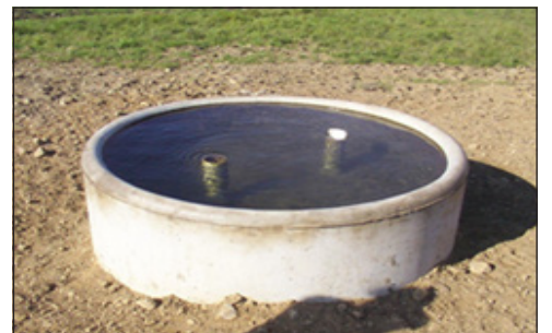
Permanent concrete water trough
